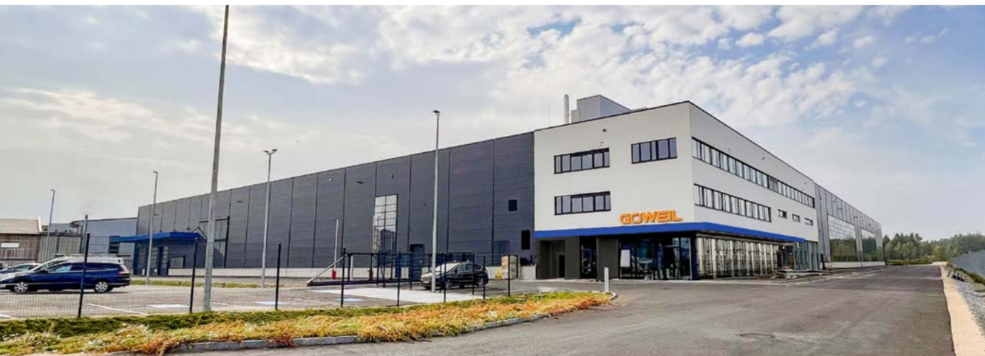
Company locations in Kirchsschlag (above) and Rainbach (below)
